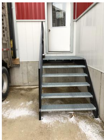
Pic 2: → Proper stairs for safety
