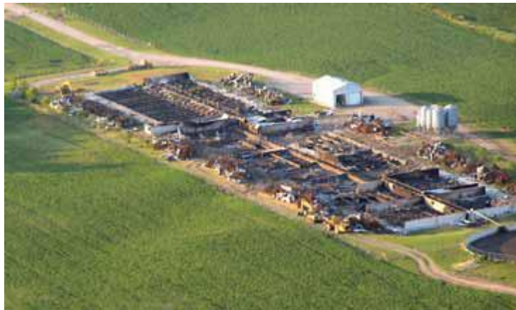
Figure 1: This large swine barn was completely destroyed by fire. (Photo credit: P. Stolk, Farm Mutual Reinsurance Plan)
